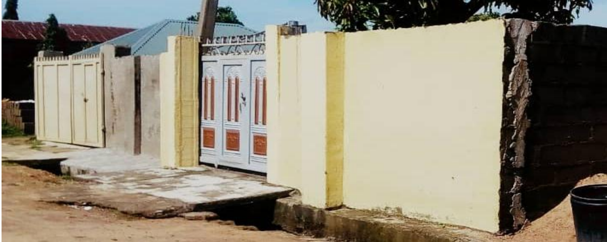
Plate 2: Building modification through fencing Source: Authors Field Survey, 2019.
