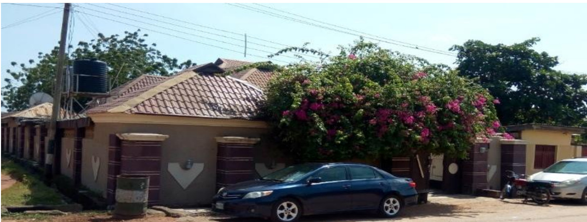
Plate 4: Building that has been completely modified from its initial design Source: Authors Field Survey, 2019.
